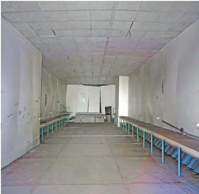
Interior of the soviet communications training bunker at Wünsdorf. Photo Clive Penfold
